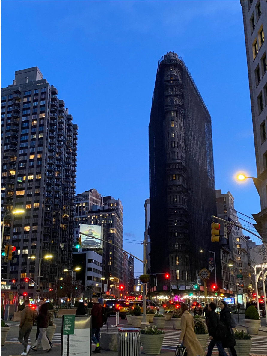
Figure 1. Shrouded Flatiron Building, New York City, USA, 2024. From author's personal collection.
